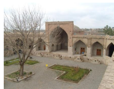
Fig 11: Picture of caravanserais after restoration (Source: Photo by the author, 2011)
